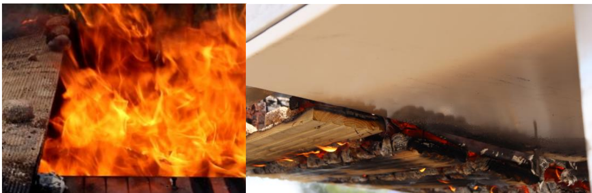
Photos showing the effects on both flammable and non-flammable soffits during the test.
